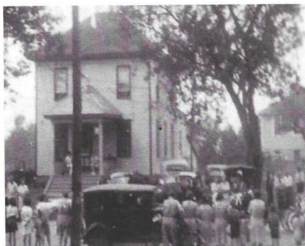
Central Office, Elgin, On. Today, it is a private home.
